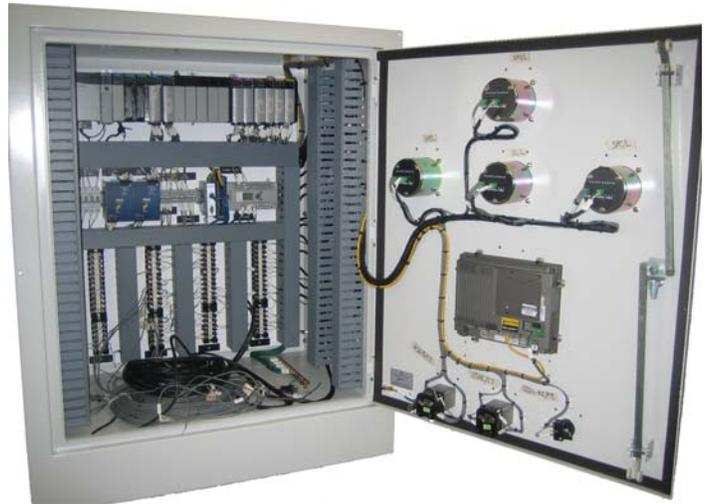
Figure 11: PLC Enclosure Cabinet - Interior
