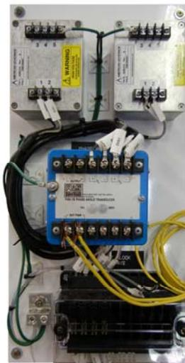
Figure 13: Voltage Phase Angle Transducer Panel
