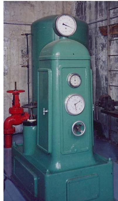
When these governors are used to control frequency or load via Speed Adjust setpoint changes (and thus not “block-loaded”) they typically cannot respond to loading variations on the grid
